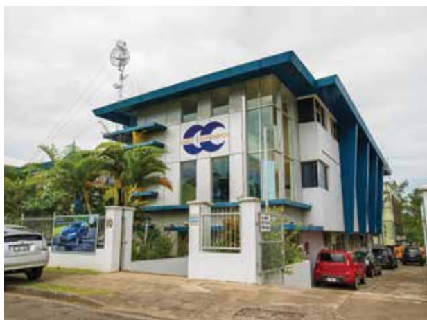
Suva Office, Fiji.
