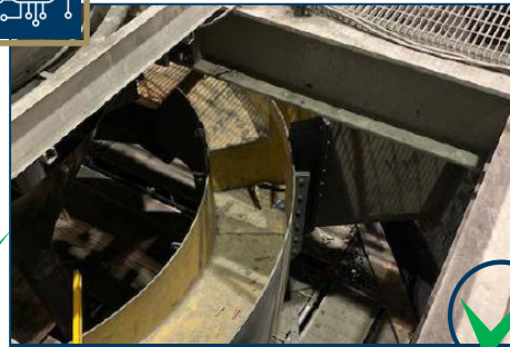
Two donut laundries installed
